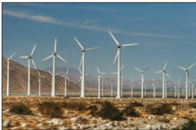
(g) Wind turbines
